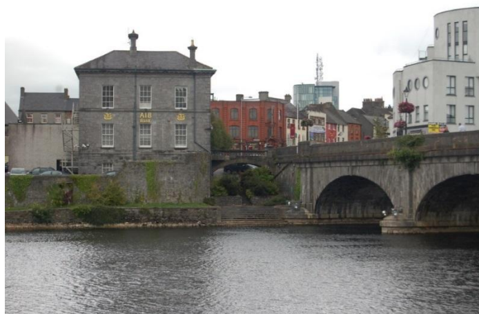
Plate 9.13 AIB Bank and Custume Bridge
