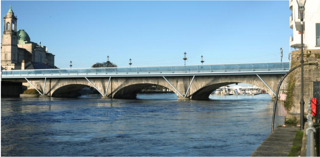
Plate 3.15 Indicative photomontage of cantilevered boardwalk attached to the south side of Custume Bridge
