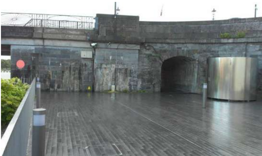
Plate 3.18 Northwest side of Custume Bridge showing the pedestrian arch
