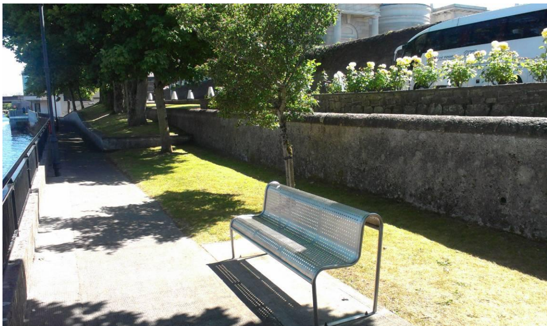
Plate 3.27 - Existing walls within the tree line
