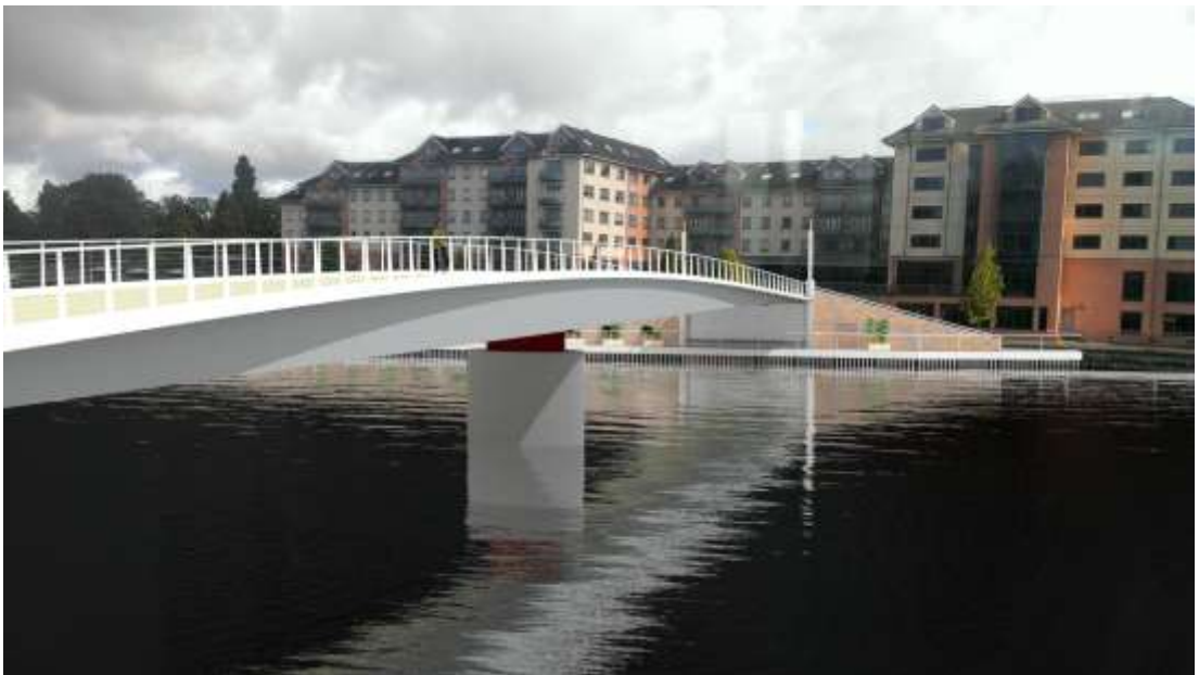
Plate 3.13 An indicative photomontage of Location 5, from the western bank, looking towards the eastern bank
