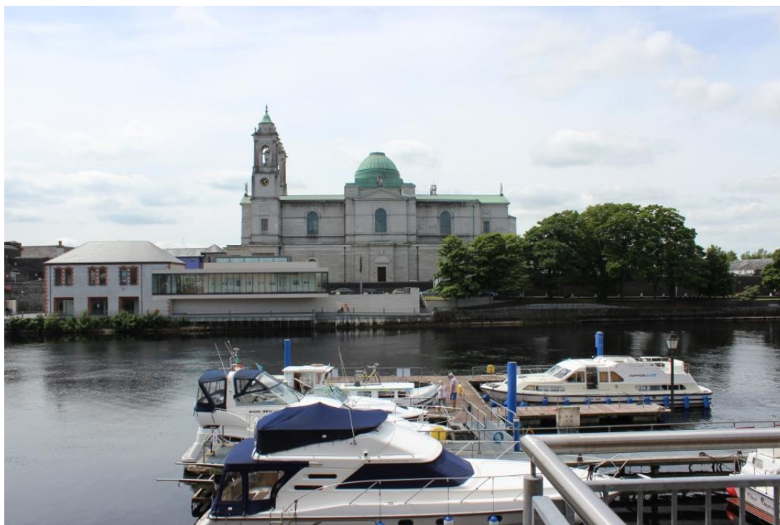
Plate 4.3 View looking west across the River Shannon from the existing marina to the Church of St. Peter and St. Paul and Luan Gallery
