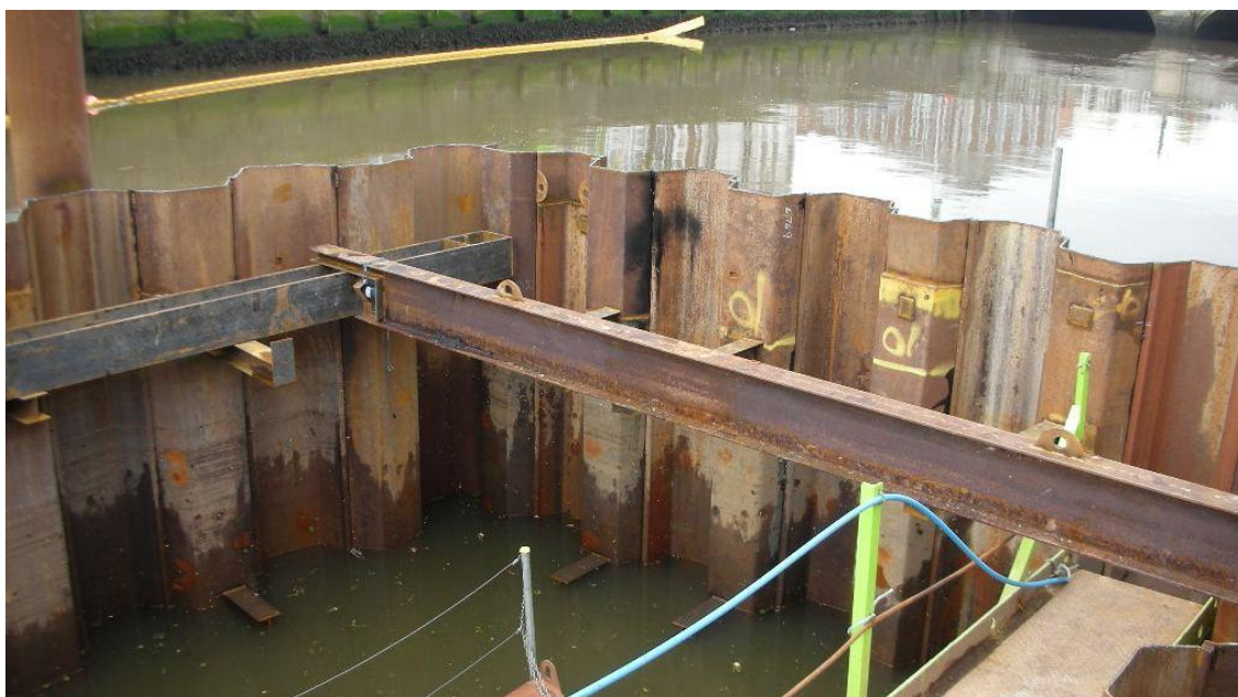
Plate 4.8 Typical cofferdam arrangement
