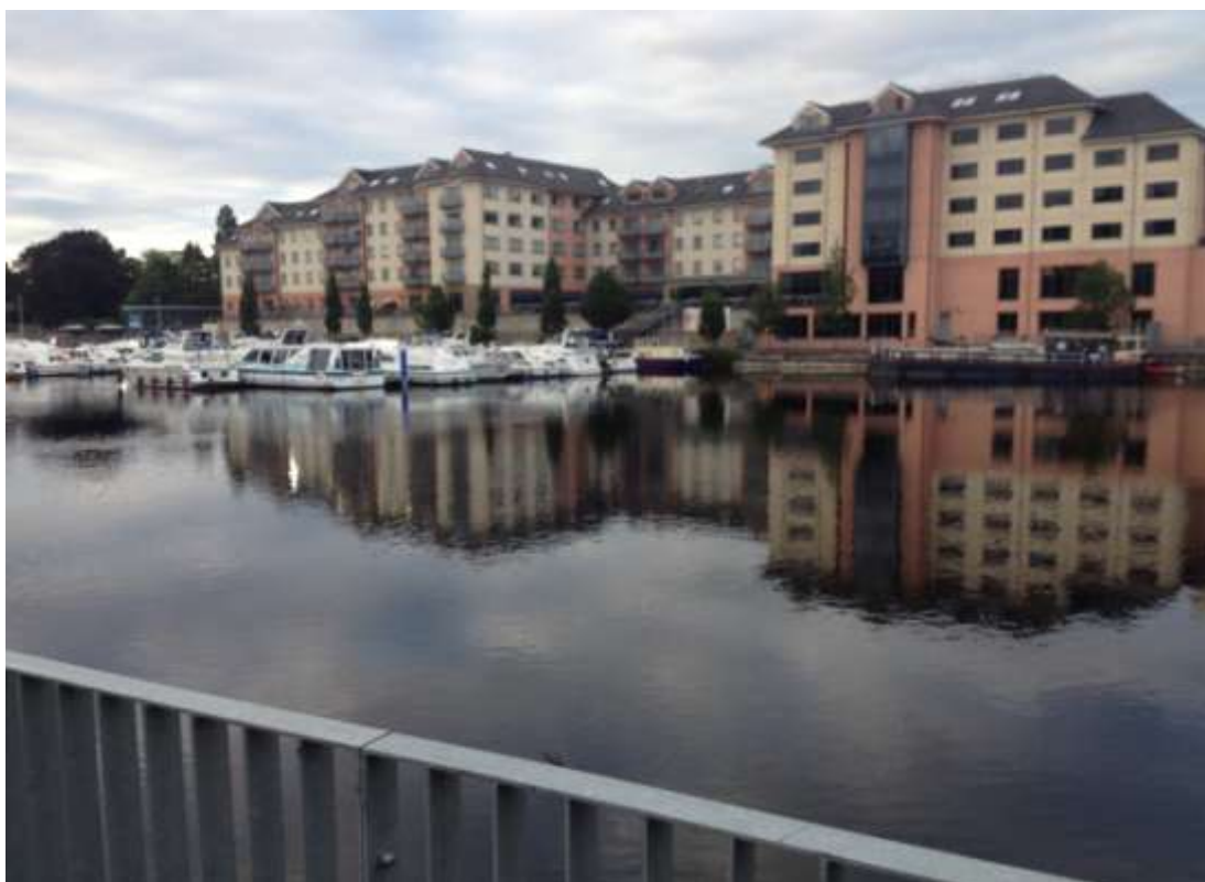
Plate 6.1 Built habitats surrounding the River Shannon at the site of the proposed development as viewed from the left (western) bank.
