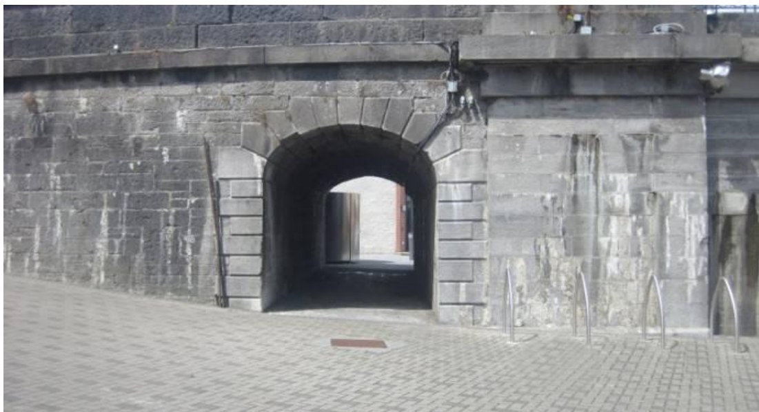
Plate 5.6 Existing bicycle parking adjacent to Custume Bridge archway
