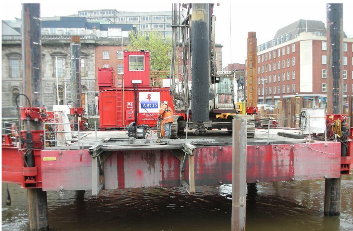
Plate 4.9 Example of Jack up barge
