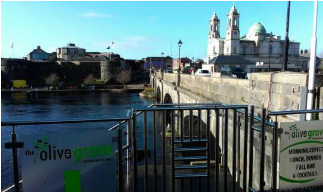
Plate 3.17 Potential east abutment location on the south side of Custume Bridge
