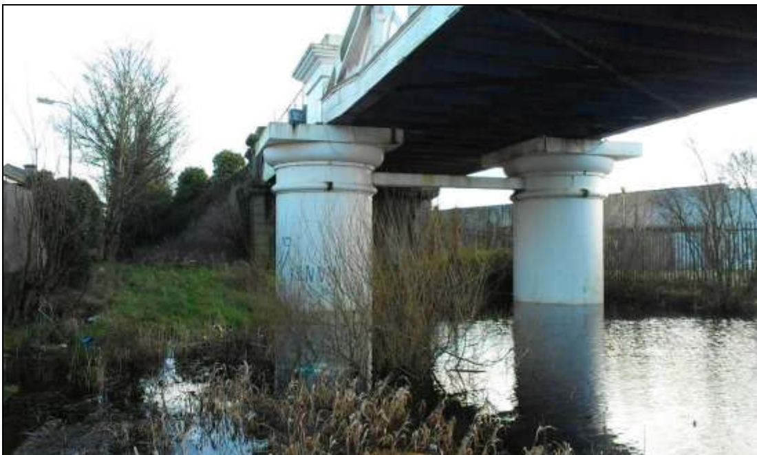
Plate 3.5 Existing piers and wing wall under the Railway Bridge
